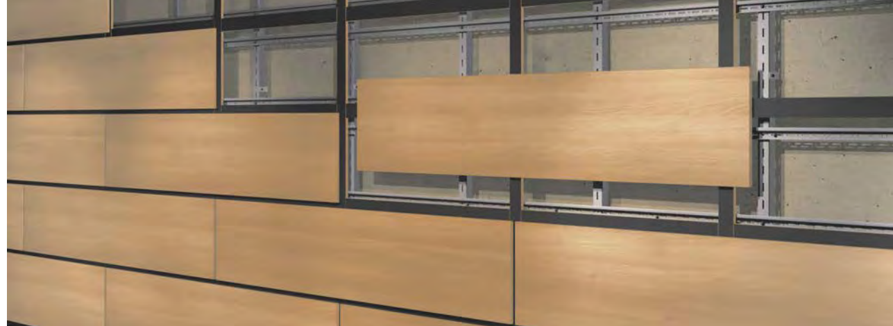
horizontal mounting with strips as joint backing (16mm thickness)
